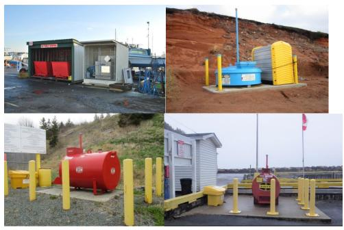
Images represent examples of outdoor used oil tank installations with proper protection from vehicle impacts (fencing, bollards).
