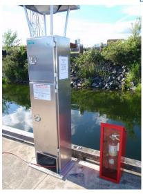
Power outlet distribution with breakers and lights fixture combined.
