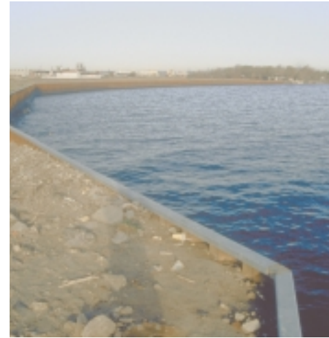
Vertical retaining walls provide little fish habitat.
