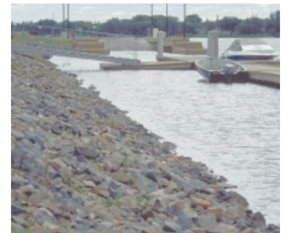
Bank stabilization using rock rubble.
