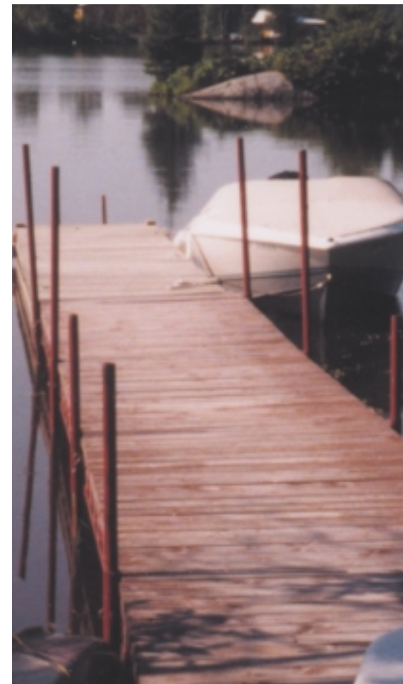
Post-supported docks cause minimal disturbance to lake or river bottoms.
