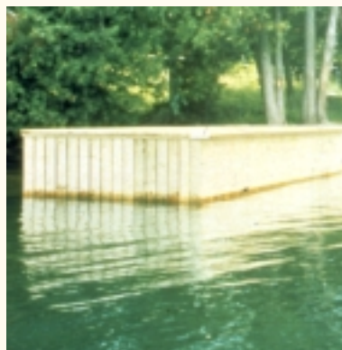
Vertical planking is not desirable.
