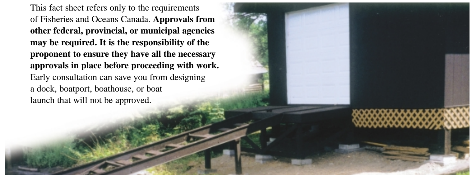
A boathouse built above the high-water level prevents damage to fish habitat.
